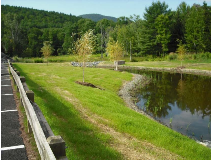
Figure 3.32 – Porous asphalt pavement and low-lying vegetation and retention pond: parking lot system
