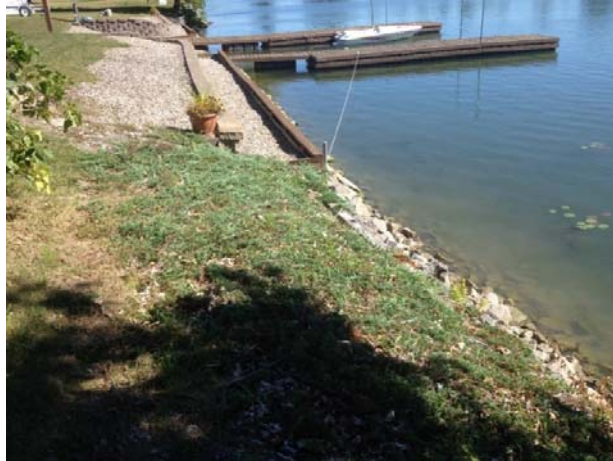
Figure 3.21 – Use of riprap and structural shore walls, as well as natural vegetative features
