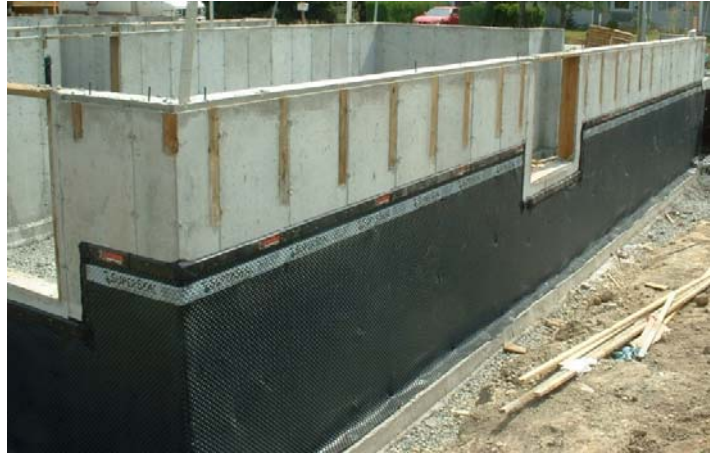
Figure 3.27 – Waterproof membrane used to protect concrete foundation (Image courtesy of SUPERSEAL Construction Projects)
