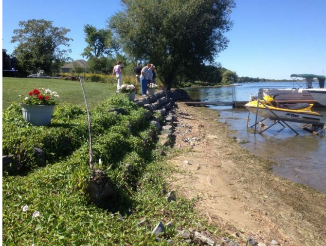
Figure 3.23 – Hard and soft mitigation combined, using limestone blocks and natural vegetation to create a resilient shoreline
