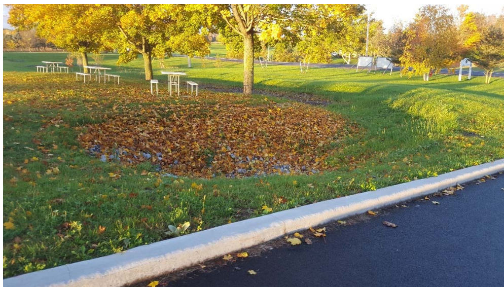
Figure 3.36 – Bioretention area for efficient use of the land and effective runoff collection
