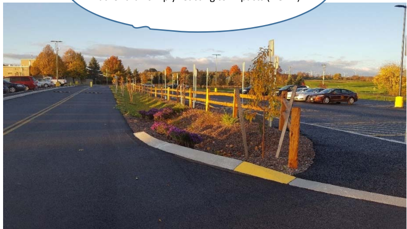
Figure 3.35 – Porous asphalt pavement and bioretention cell to reduce impervious surfaces and make a parking lot area more sustainable
