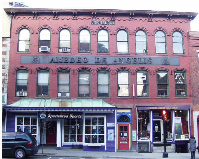
Photo: Main Street, Union Block by Ken Gallager / CC BY-SA 2.0
