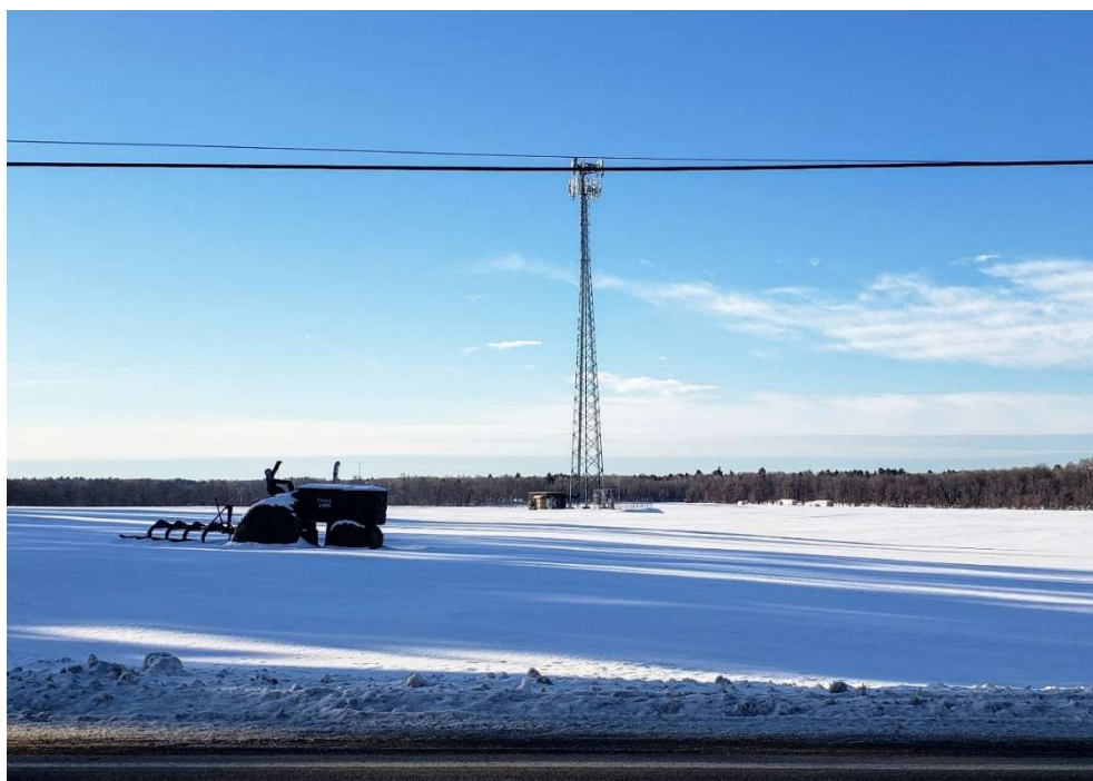
FIGURE 8 LATTICE TOWER WITH TWO LEVELS OF CELLULAR ANTENNAS.
